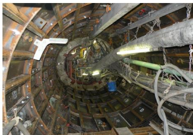
Secondary Lining in progress
